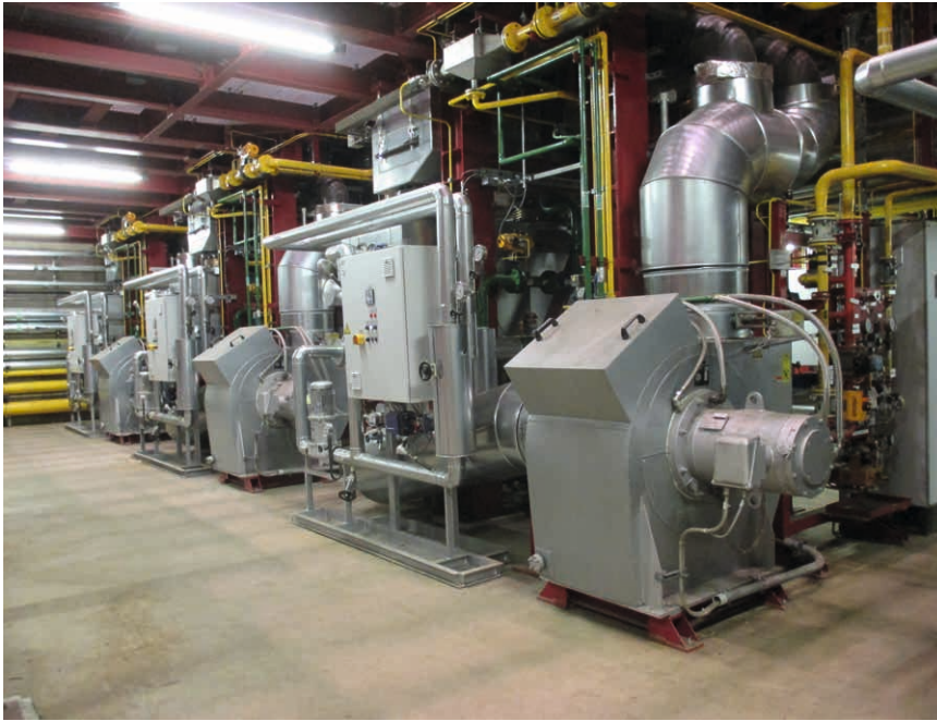
The LOI-developed bypass cooling system featuring dual coolers has been installed in the basement
